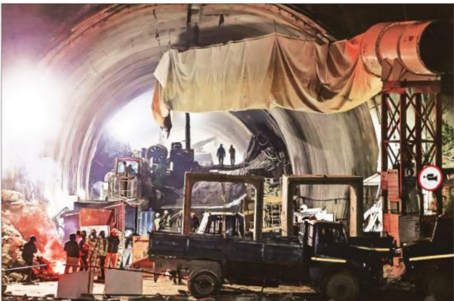
The rescue operation in progress at the Silkyara-Barkot tunnel in Uttarakhand on Monday.
