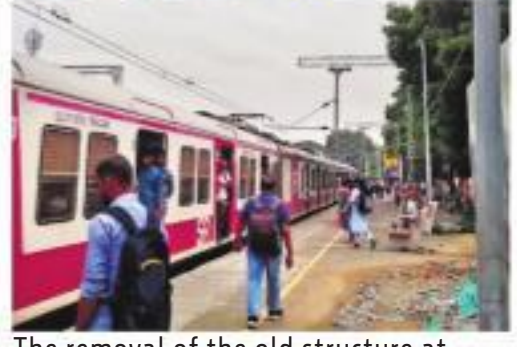
The removal of the old structure at the station has brought much relief to passengers | EXPRESS / JOSLIN MARIAM JOHN
