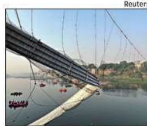
The Morbi suspension footbridge collapsed last year killing 135
