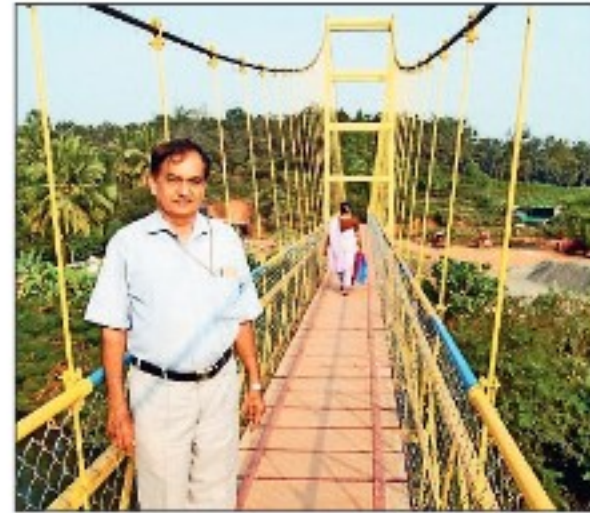
Bharadwaj built over 140 hanging footbridges connecting villages separated by rivers
