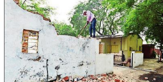
Demolition started from Abhay Ghat for renovation of the Gandhi Ashram in Ahmedabad on December 23, 2021
