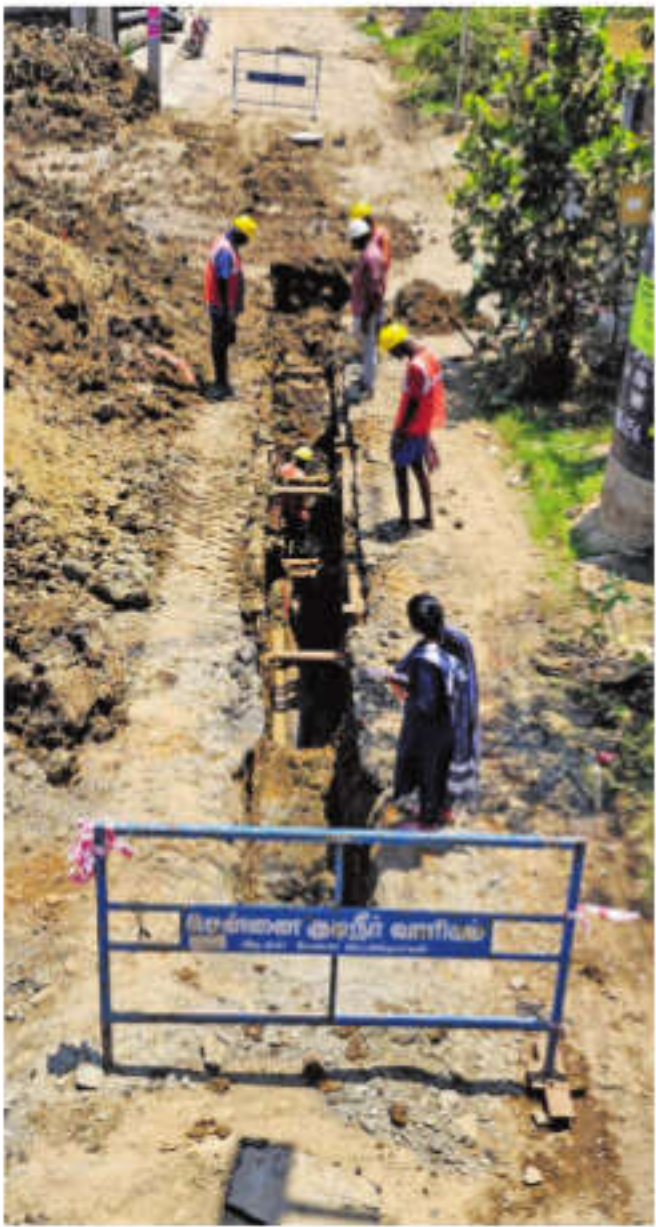
Roads were dug up for the UGD work in Madipakkam area in the city | EXPRESS
