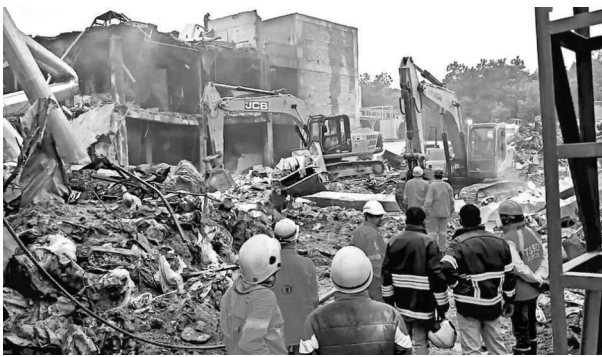
Fire and rescue personnel during a rescue operation in Sangareddy district, Telangana, on Tuesday. P77
