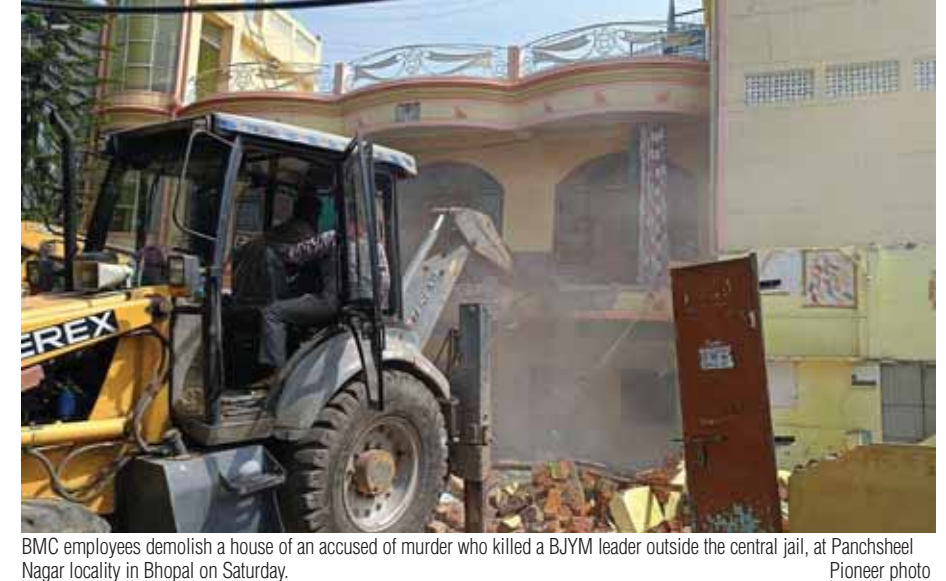
BMC employees demolish a house of an accused of murder who killed a BJYM leader outside the central jail, at Panchsheel Nagar locality in Bhopal on Saturday. Pioneer photo
