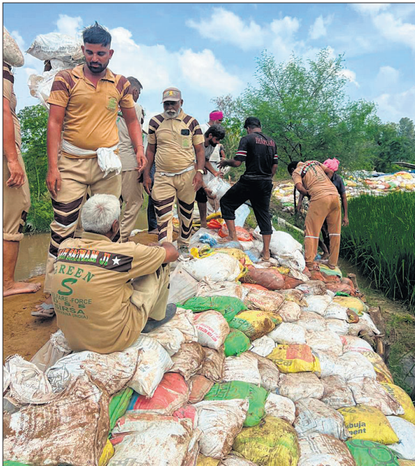
Banks of the Ghaggar being strengthened by volunteers at Rattakhera village. TRIBUNE PHOTO
