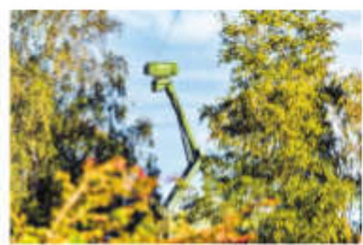
A mobile radar installation at Denmark's Pionegaarden military site near Dragør on the Øresund coast, overlooking the sea between Sweden | AP
