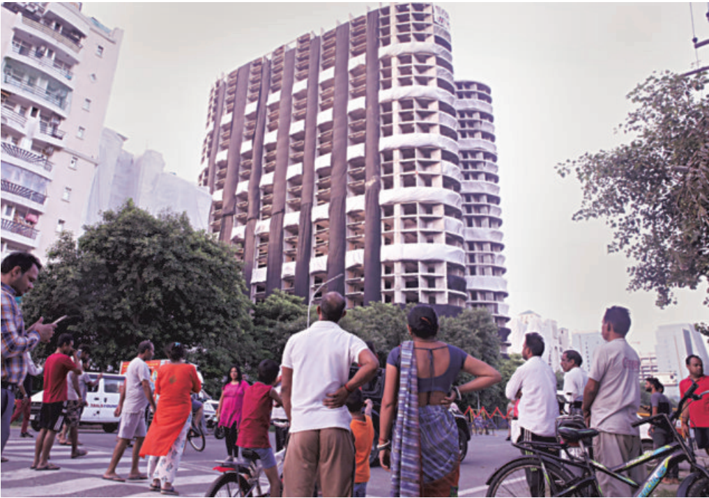
The dust settled in an hour, but it will take 90 days to clear the 12,867 cubic metres of debris
