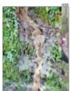
NOT AGAIN: Residents spotted muddy water spouting from the hillside on Sunday morning.
