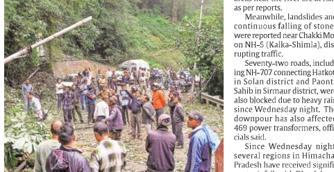
Workers clear a road that was blocked by an uprooted tree following heavy rainfall, in Shimla, Thursday.
